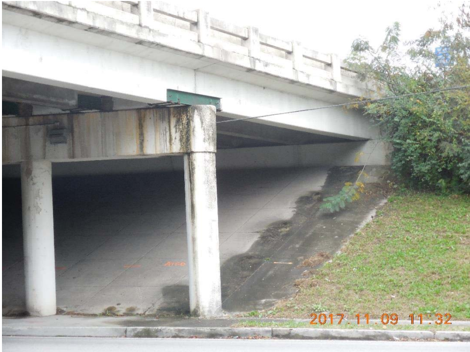
Looking at Abutment No. 1
