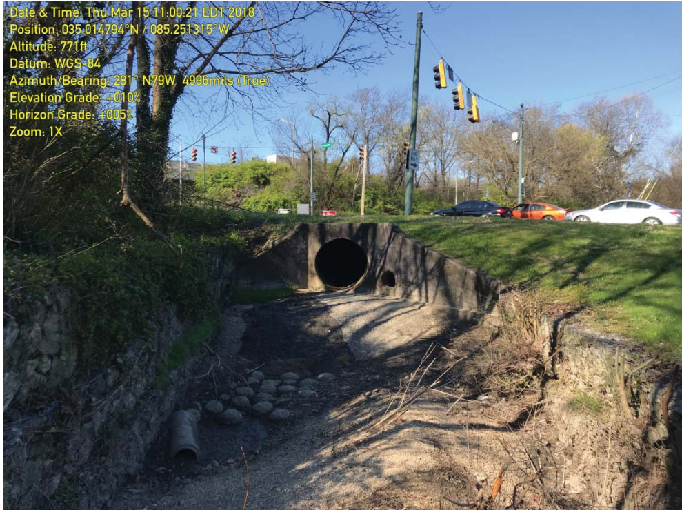
Photograph 1 – IMG_2707 - View of STR-1 looking upstream at culvert outlet, this culvert conveys the stream under the I-24 / Germantown Road intersection
