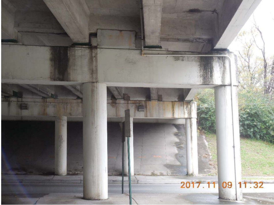
Looking at Bents No. 1 and No. 2
