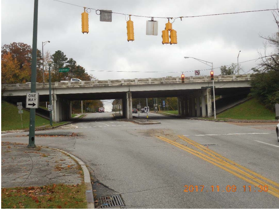
Looking South under Bridge
