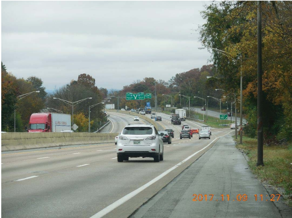
Looking East over Bridge
