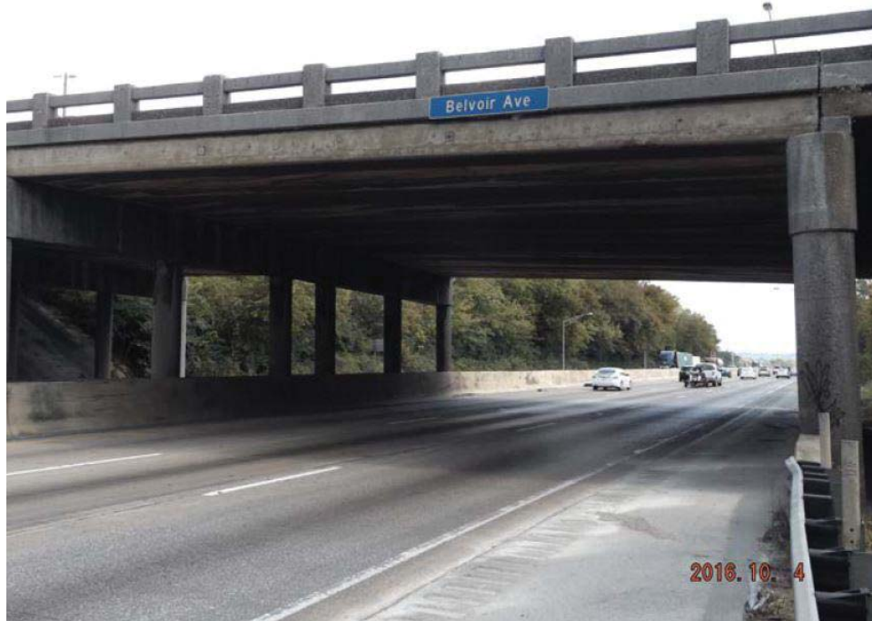
Bottom of Deck / Clearance - Eastbound
