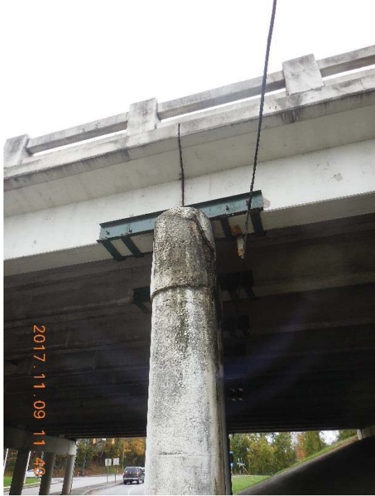
Looking at North at Bent No. 3
