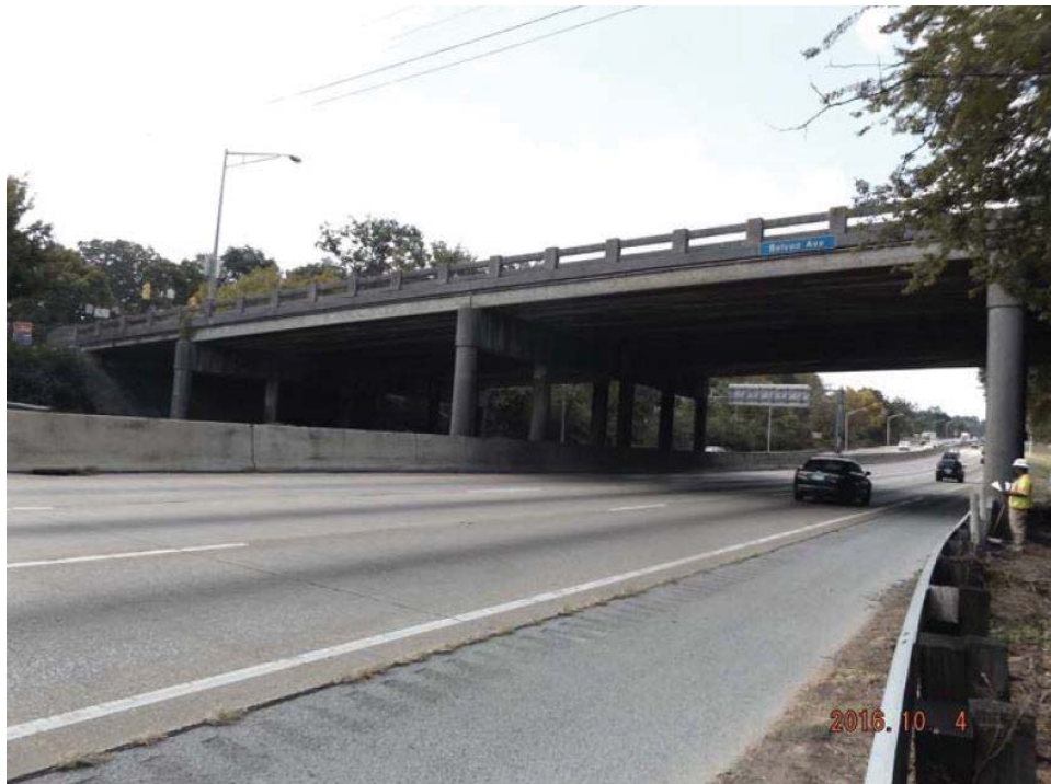
Bottom of Deck / Clearance – Westbound (Right Side)
