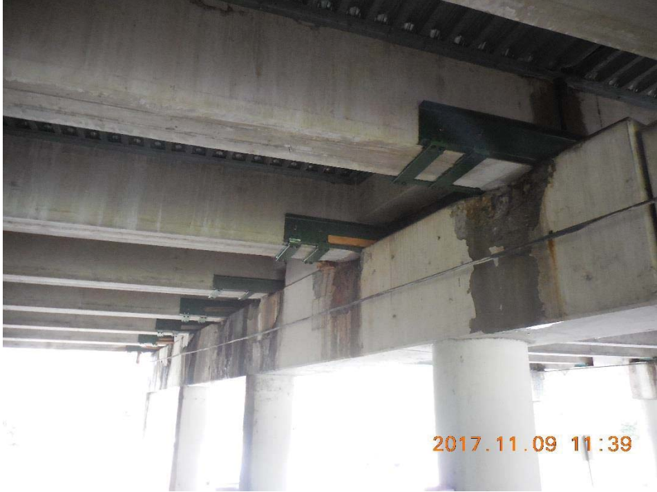
Looking at Bent and Beam Supports
