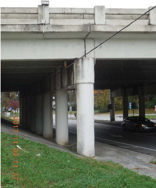
Looking at Bent No. 1
