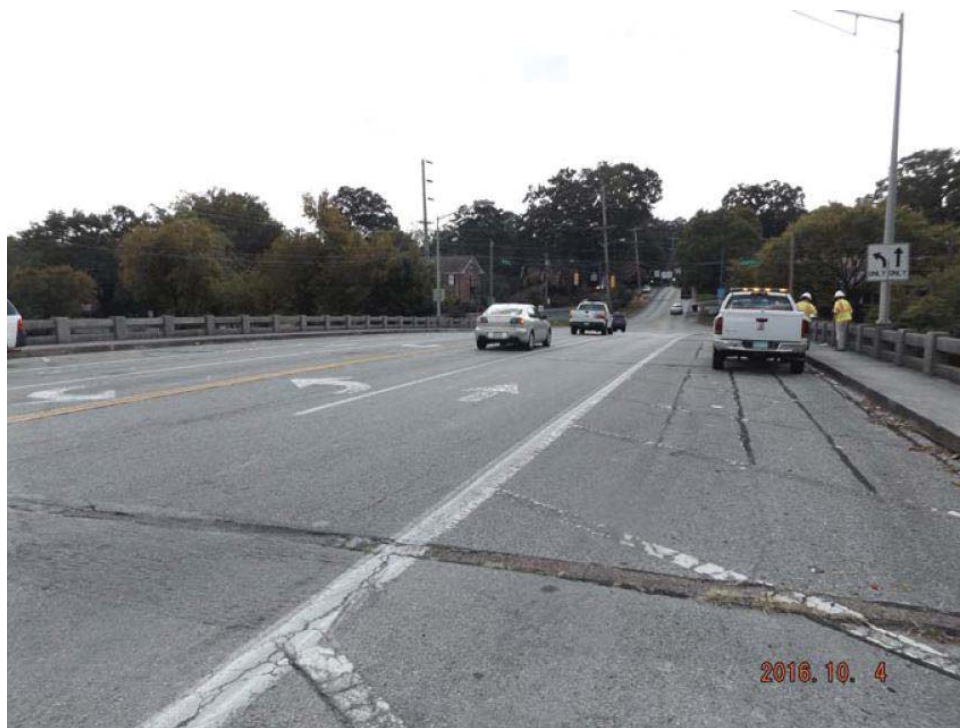
Top of Deck - Southbound
