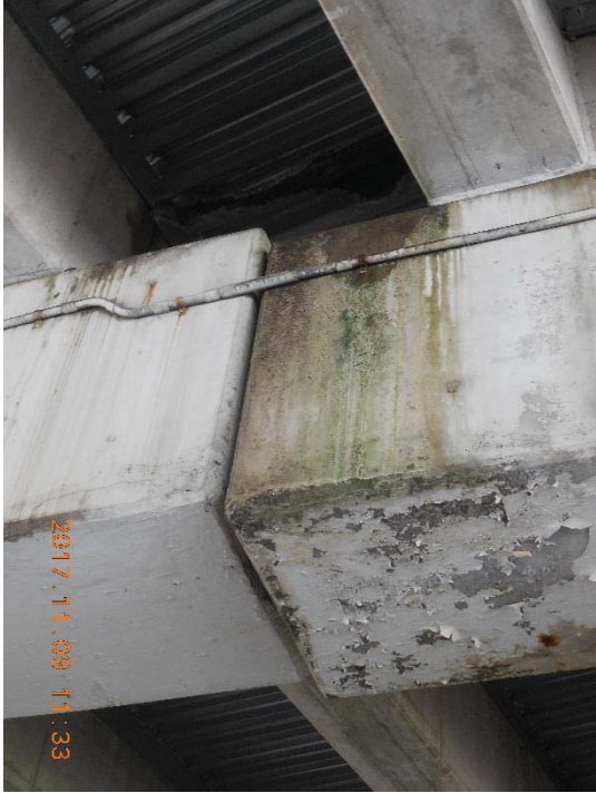
Widened Bent Caps
