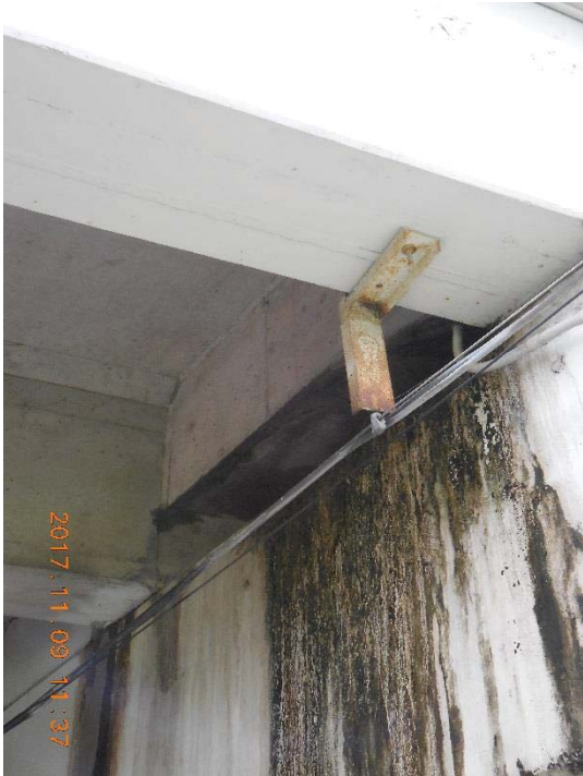
Utilities Mounted to Bridge
