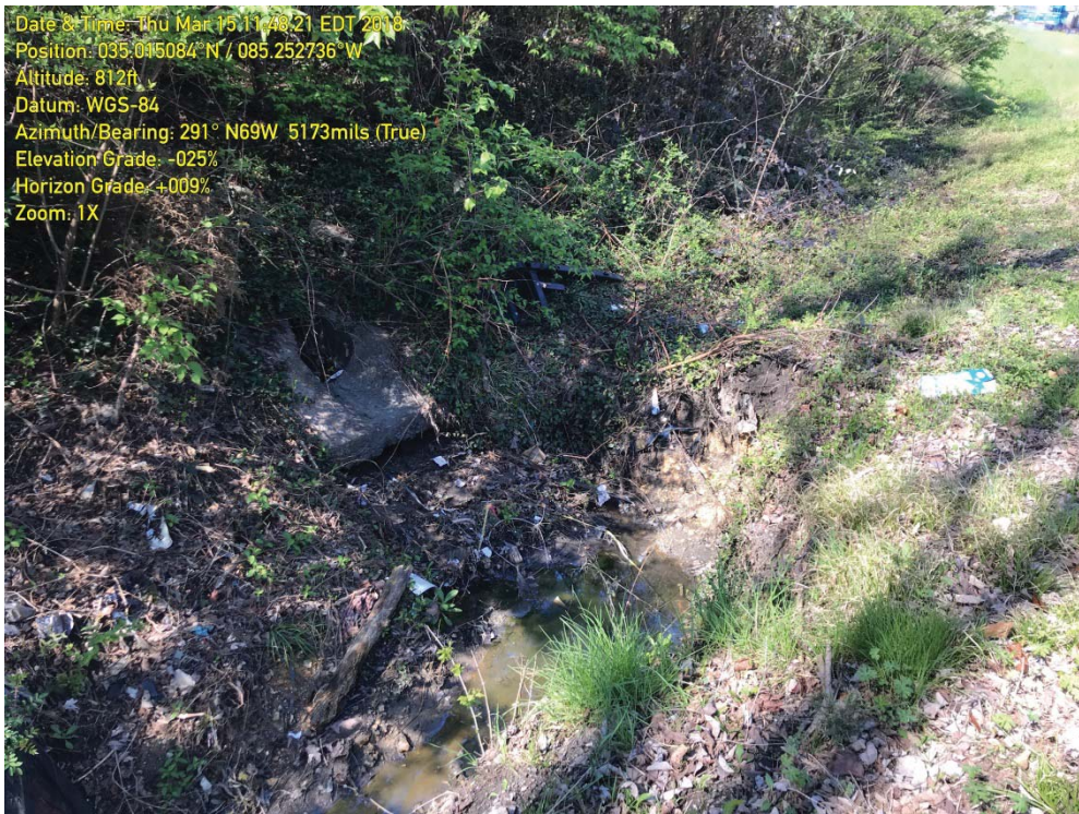
Photograph 8 – IMG_2728 - View of STR-2 looking upstream at the origin between I-24 west and the I-24 west entrance ramp
