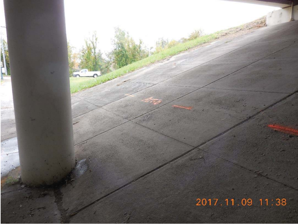
Concrete Slope Paving
