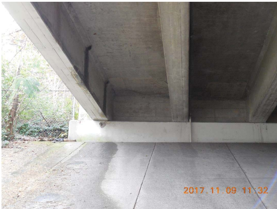
Looking at Abutment No. 2
