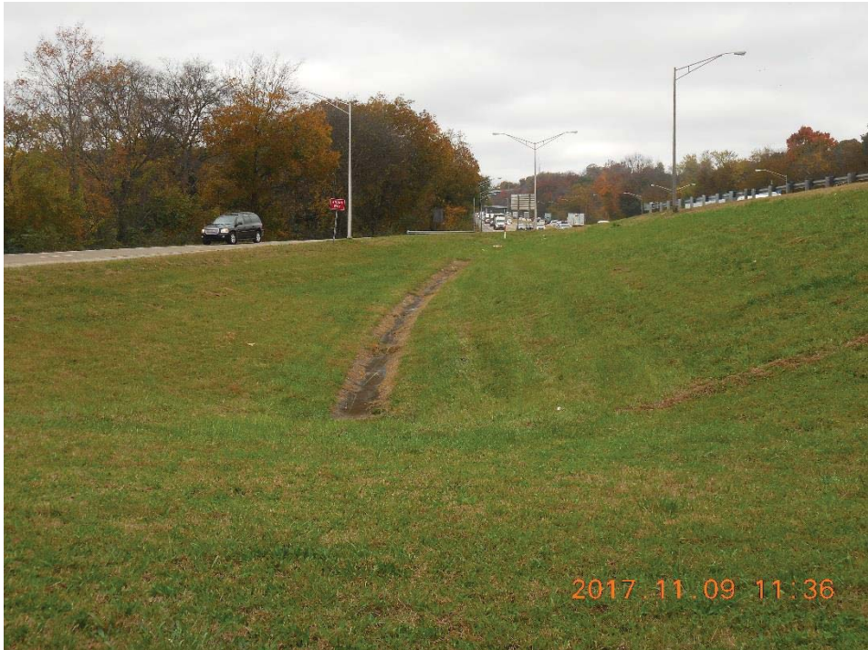
Drain at Southwest side of Bridge
