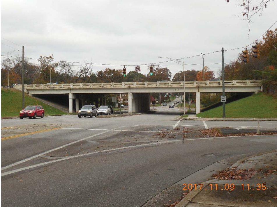
Looking North under the Bridge
