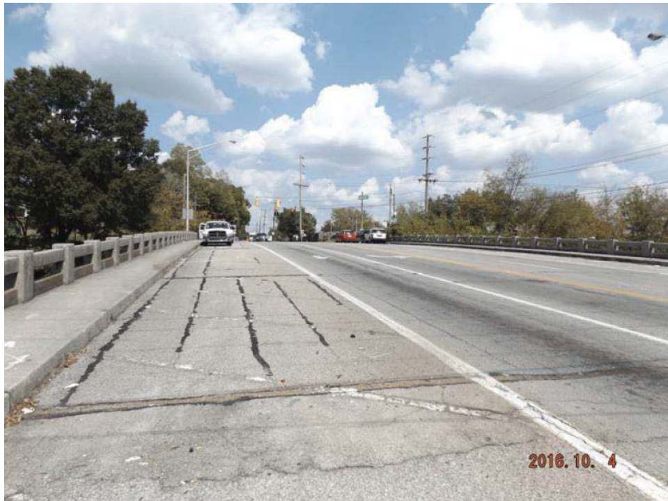
Top of Deck - Northbound
