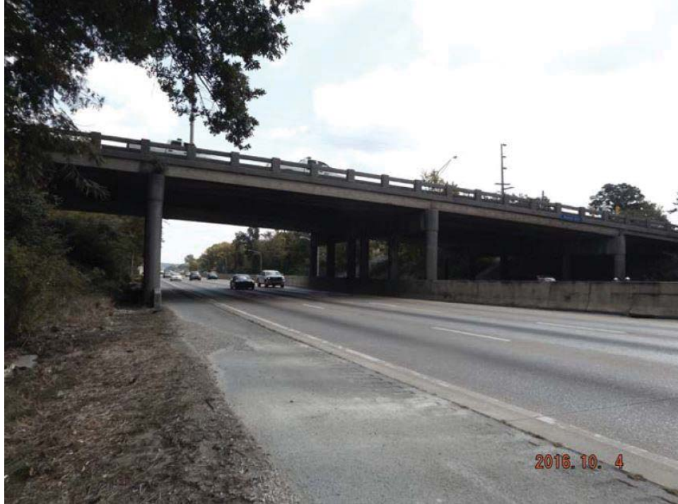
Bottom of Deck / Clearance – Westbound (Left Side)
