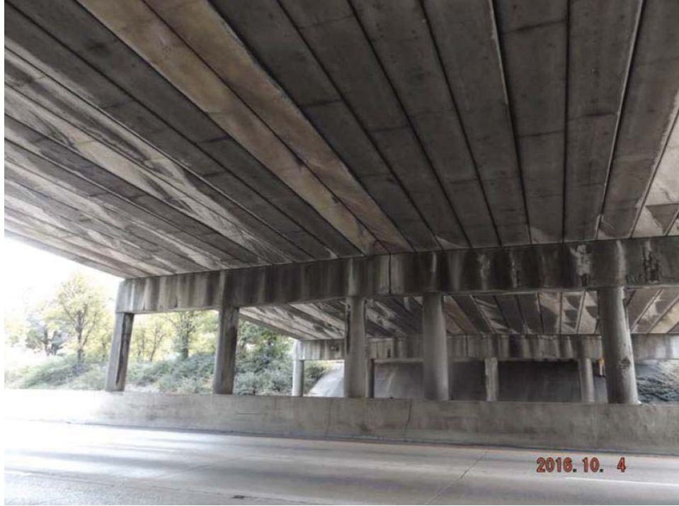
Span No. 3 / Bent No. 2
