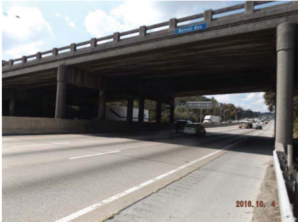
Bottom of Deck / Clearance – Westbound
