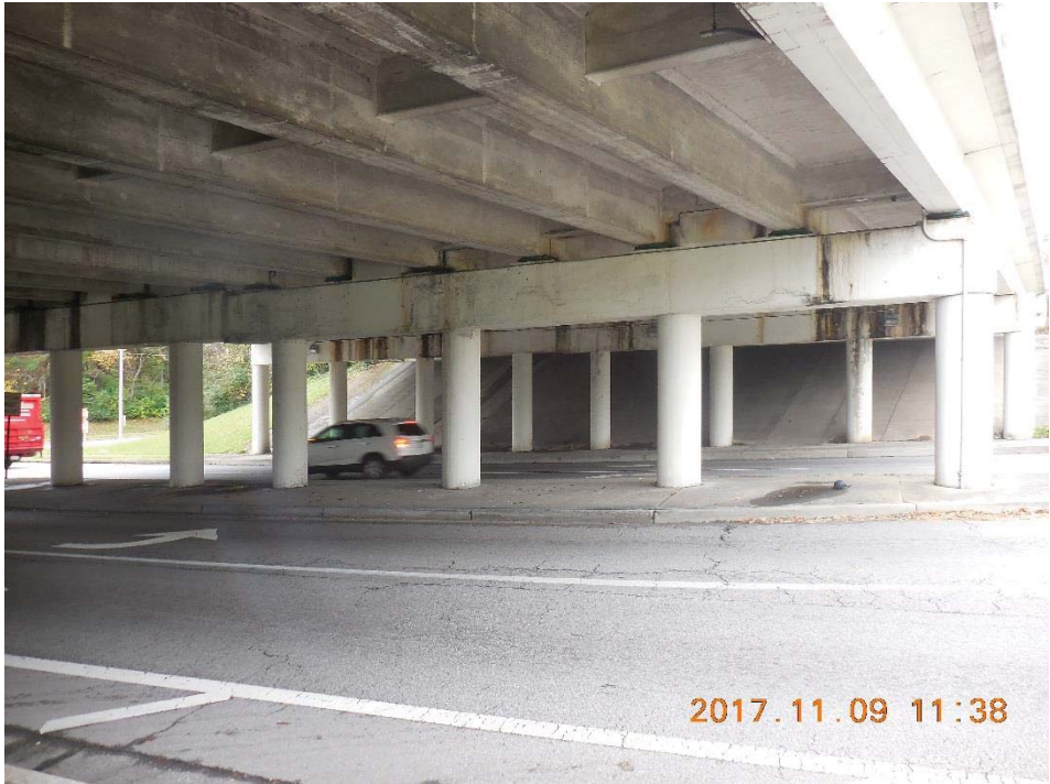
Looking under Bridge at Bents
