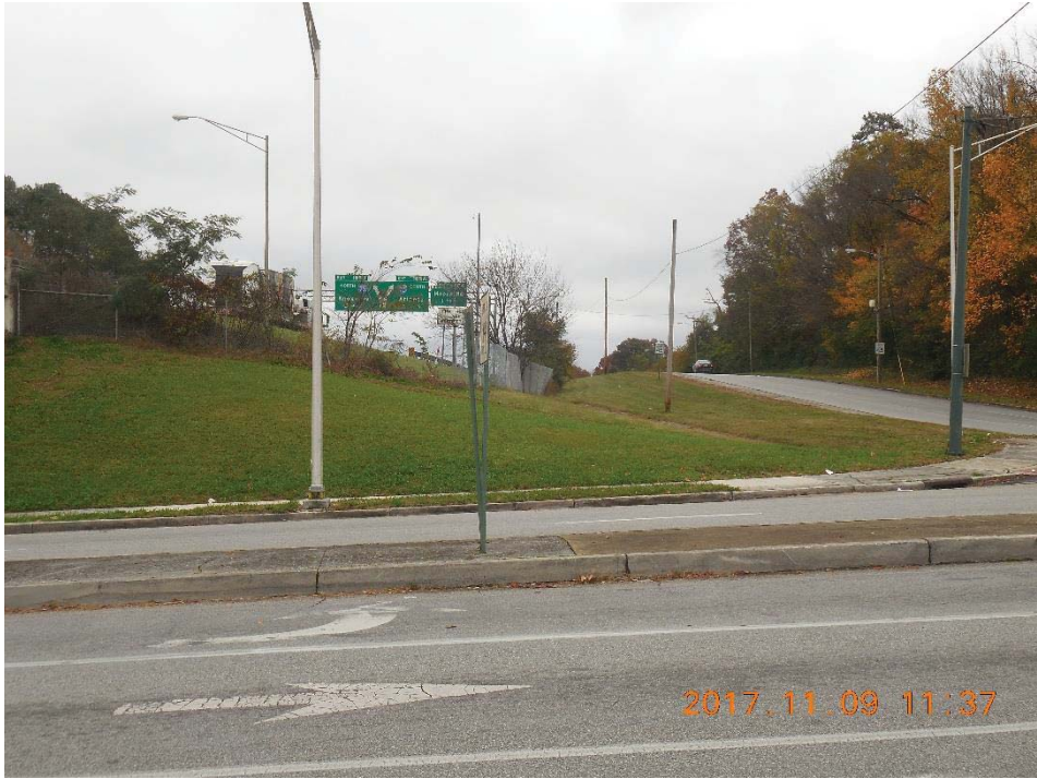
Looking East at On-Ramp
