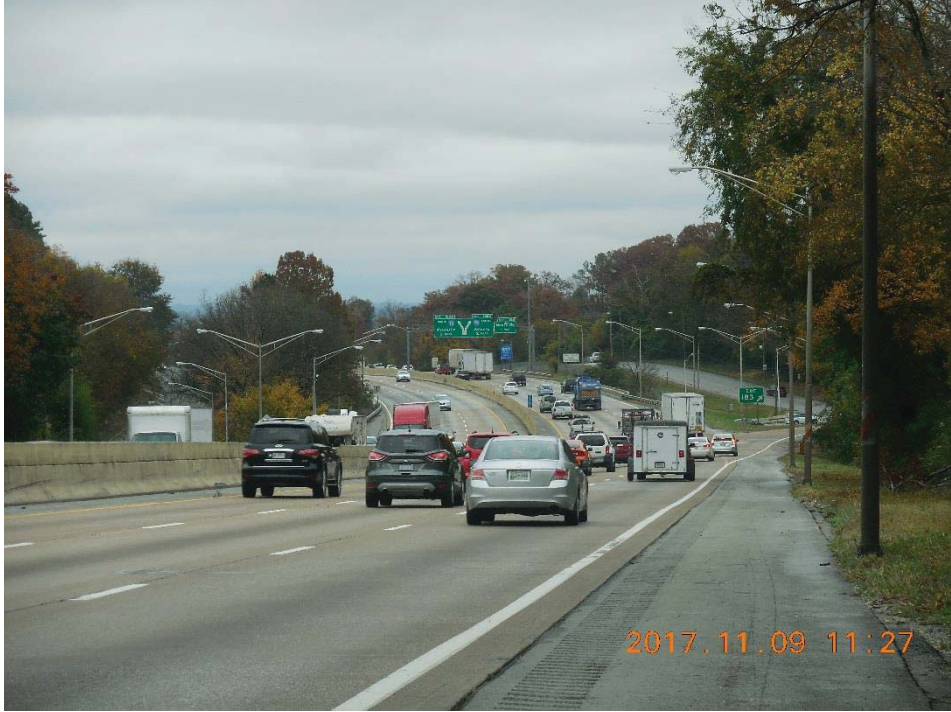
Looking East over Bridge
