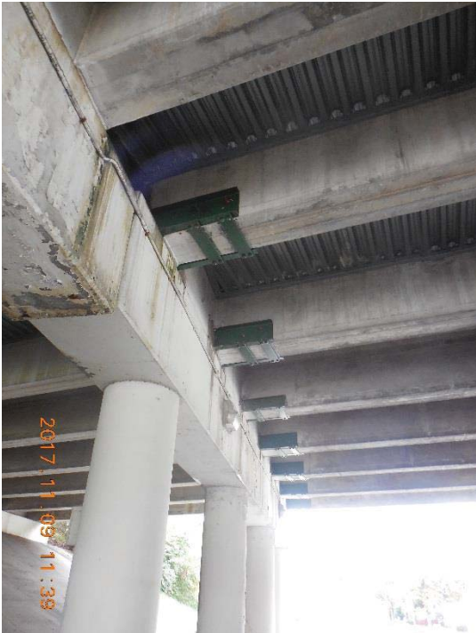
Looking at Underside of Deck
