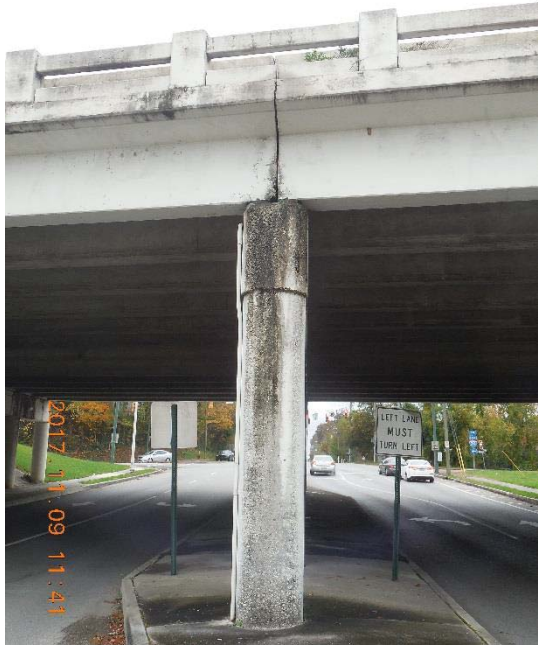
Looking North at Bent No. 2
