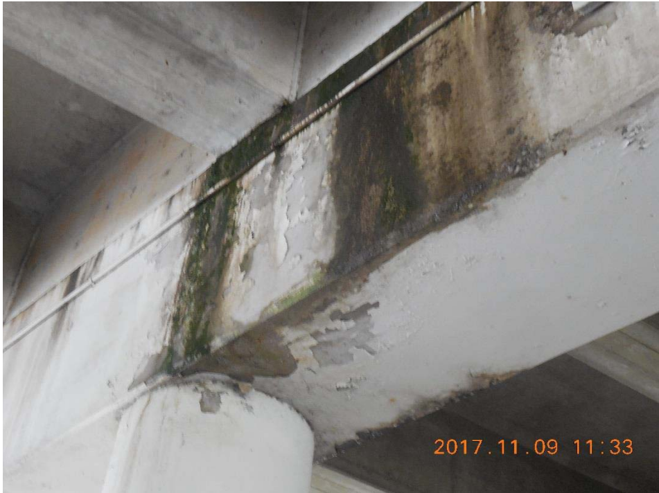
Underside of Bent Cap
