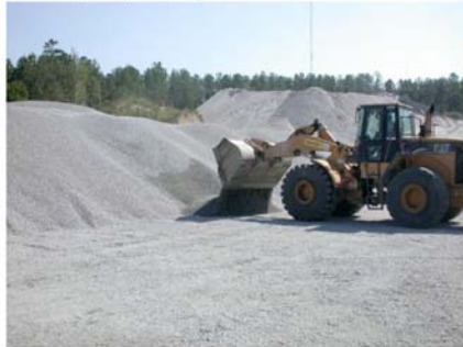
Step 2. Loader gently rolls the material out of the bucket to form a small pile
